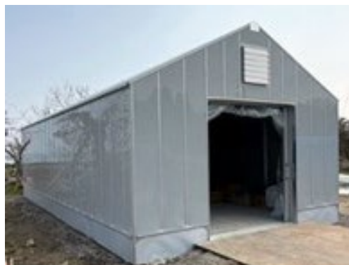
Building housing the CO 2 electrolysis system installed at the demonstration site in Suzu City
