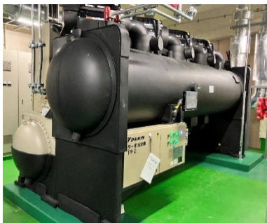
Turbo refrigerator x 1
