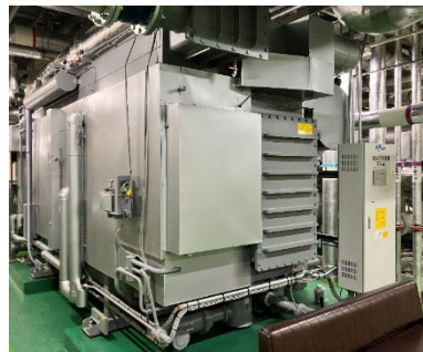
Absorption chiller x 1 unit
