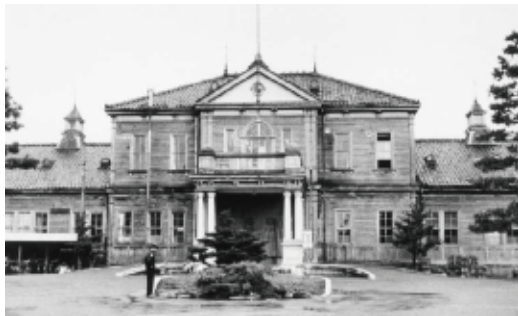
Original University Hospital building
