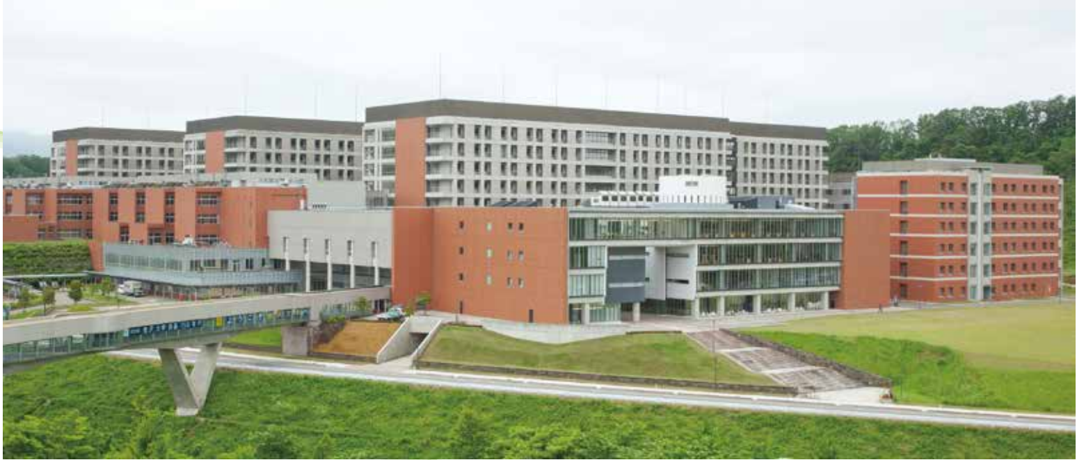
Natural Science and Technology buildings, South Area
