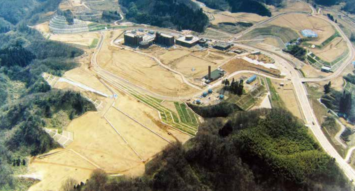
Kakuma Campus under construction (1988)
