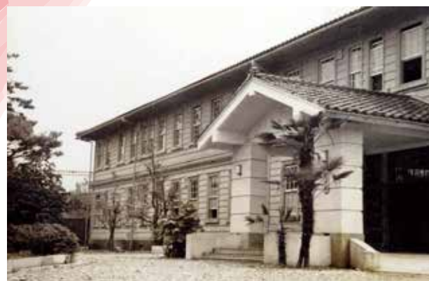
Faculty of Education buildings converted from the former Ninth Division army base
