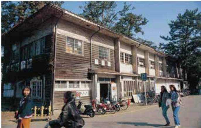
Cultural Clubs Building in the castle campus
